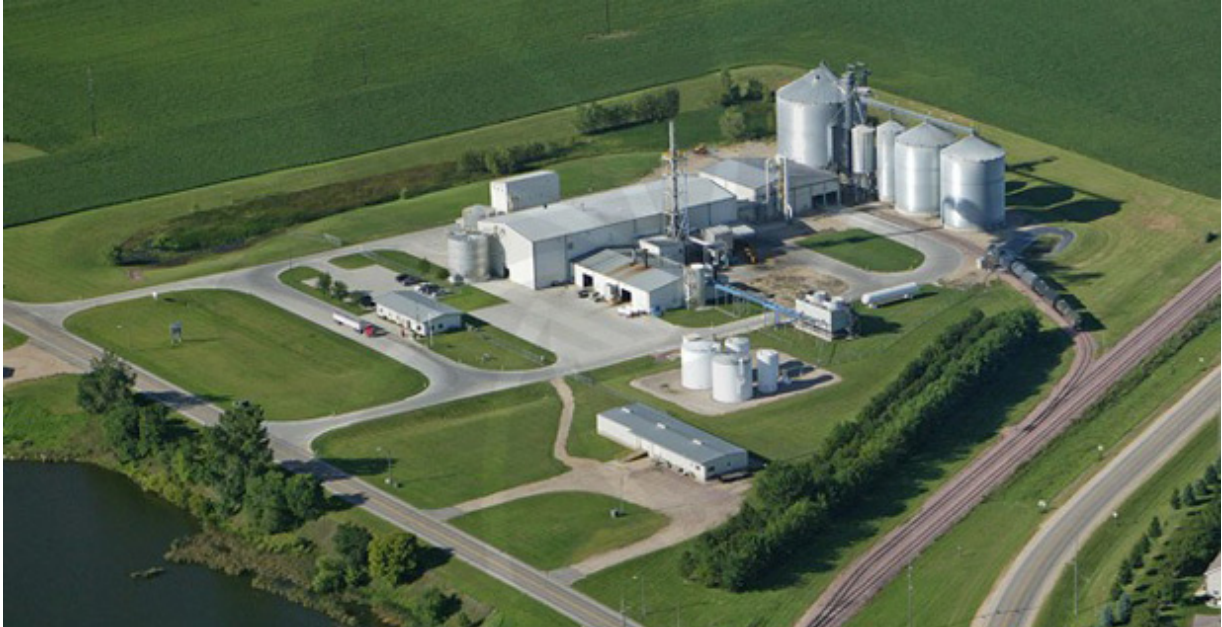
Plan B: The plant Gevo is retrofitting in Luverne, Minnesota.
